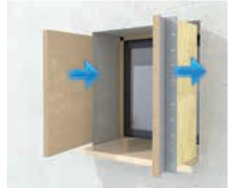
3 Install the reveals and head
